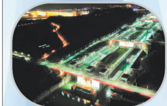
三峡南线船闸恢复通航
