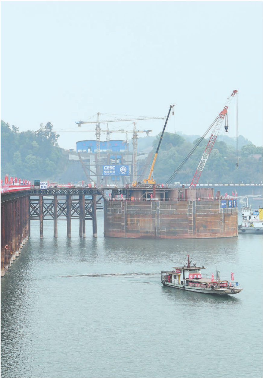
泸州长江六桥主墩钢围堰封底
