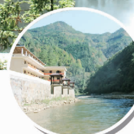
芭蕉园电站大坝下游
