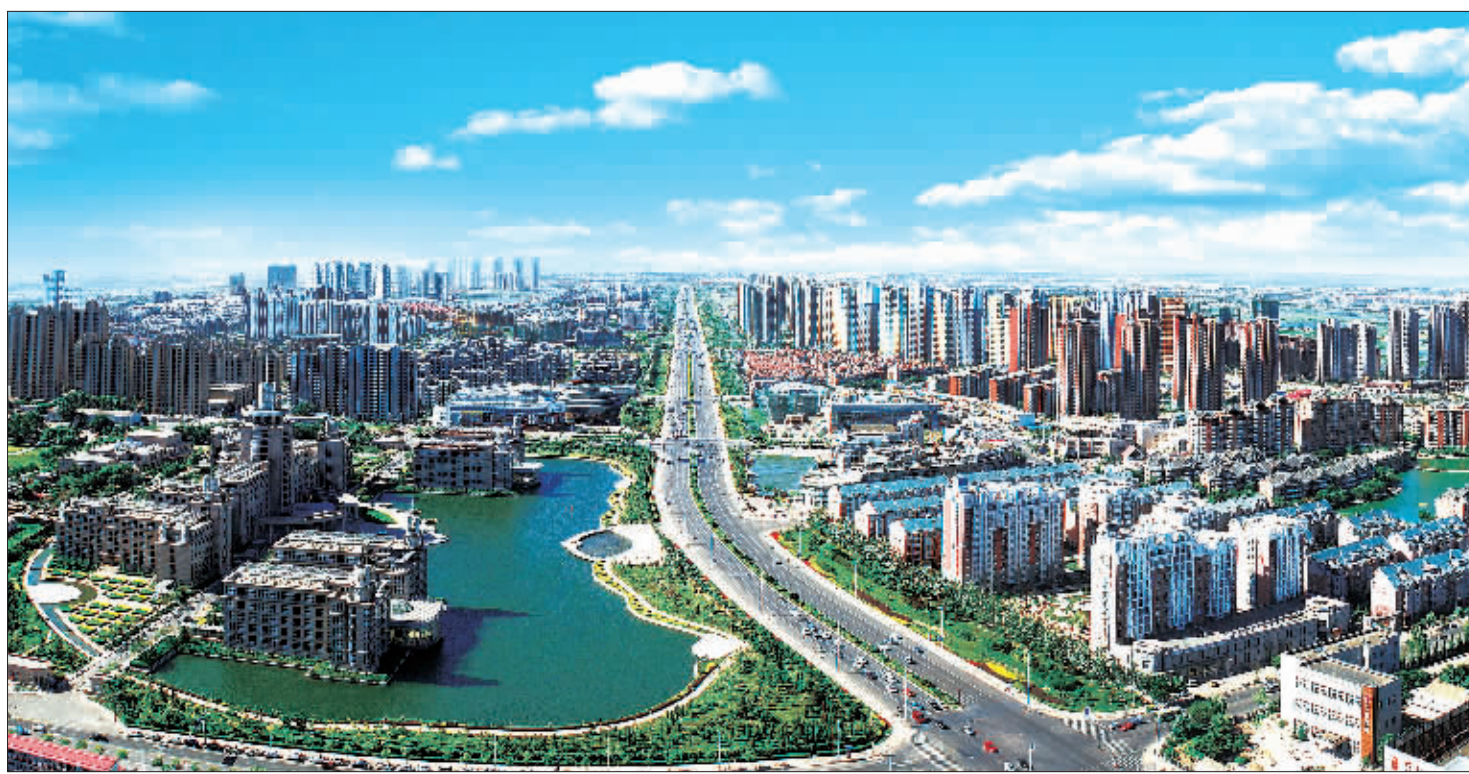
Bird's-eye view of Tianjin Meijiang Convention Center
